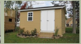
HANDI SHED WITH SIDE DOOR AND WINDOW AND A PRESSURE TREATED RAMP
